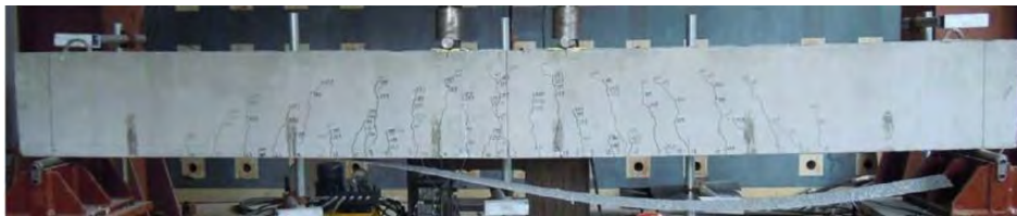
Fig.10 Failure mode of experiment for the four-point test-B [44]
