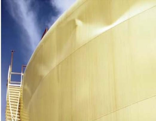
**Figure 3. Sloshing damage to upper shell of tank (courtesy of UC Berkeley)**
