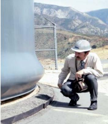
**Figure 4. Elephant-foot buckling of tank wall (courtesy of UC Berkeley)**
